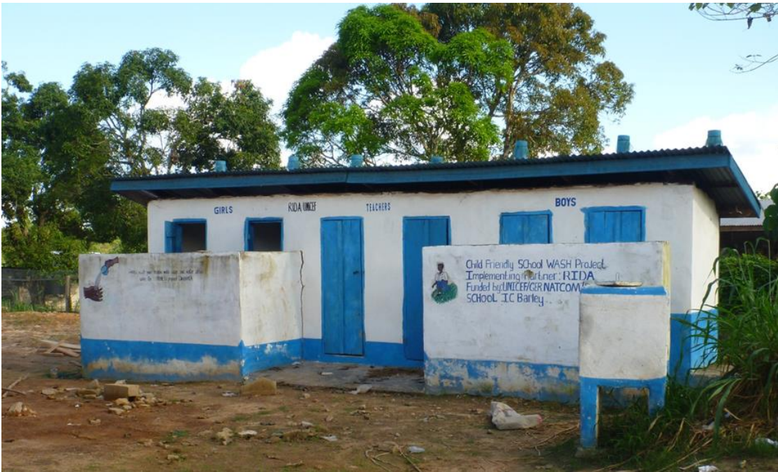
Figure 6 School VIP latrine block with six stalls.
