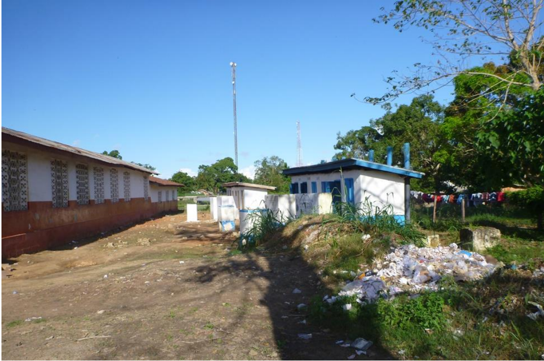
Figure 5 J.C. Barlee and TWI VIP latrines located behind the school classrooms.
